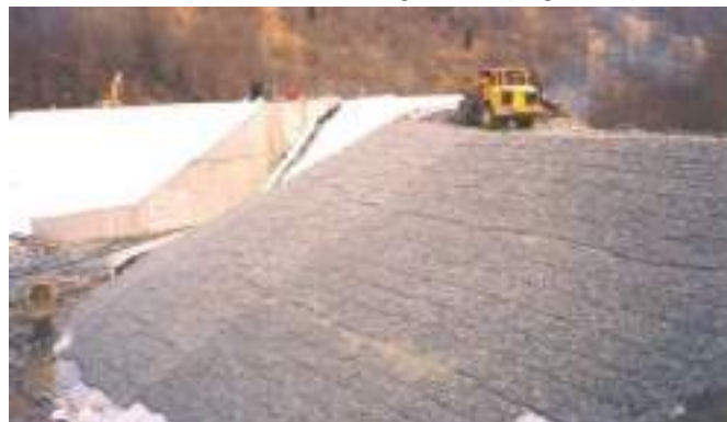
Figure n°15 : Installation de matelas Reno anti batillage
