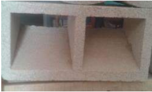
Figure 24 : Ventilation haute (VH)
