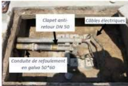
Figure 43 : Clapet anti retour
