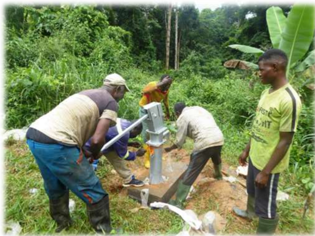
FORAGE VILLAGE DE ZOASSEL, installation de la PMH, 08/2022
