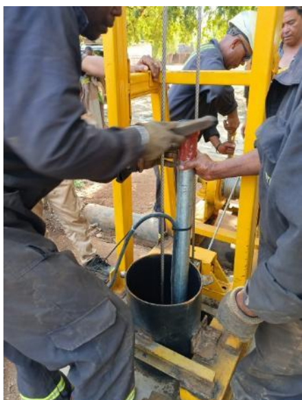
Figure V-2 : raccordement des raccord-unions
