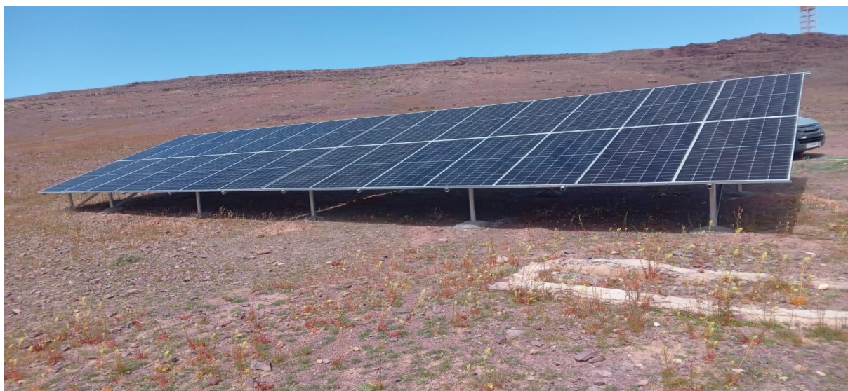
Figure 15 Installation des panneaux photovoltaïques
