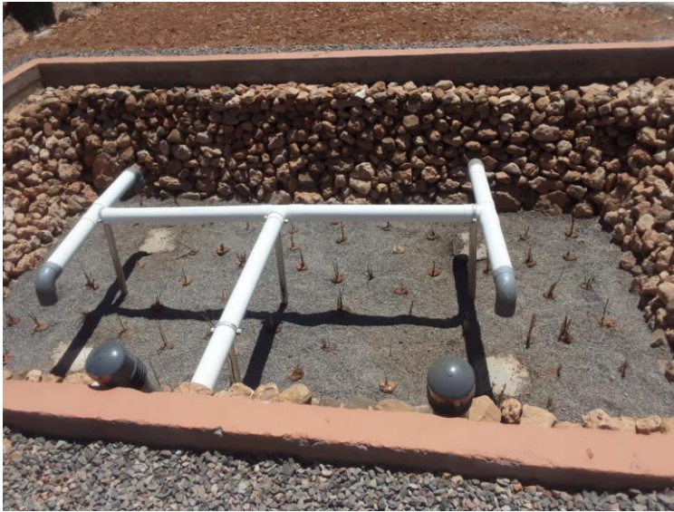
Figure 16 Fourniture et installation des roseaux
